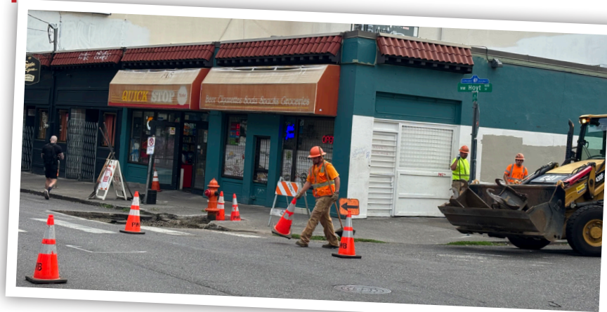
ADA ramps are being installed along Northwest 21st and 23rd avenues. The Portland Bureau of Transportation reports an average cost of ramps at nearly $250,000 for the four corners of one intersection.
