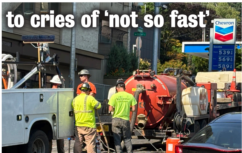
Intersection improvements at the St. Clair and Burnside intersection are under construction.
