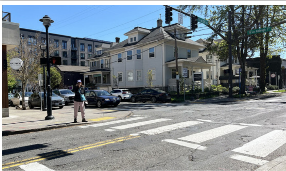
Rutted Northwest 23rd Avenue was recoated last month, a temporary fix expected to last no more than seven years. Permanent rebuilding is tied to a federal grant application to install streetcar tracks on both lanes of the street.
