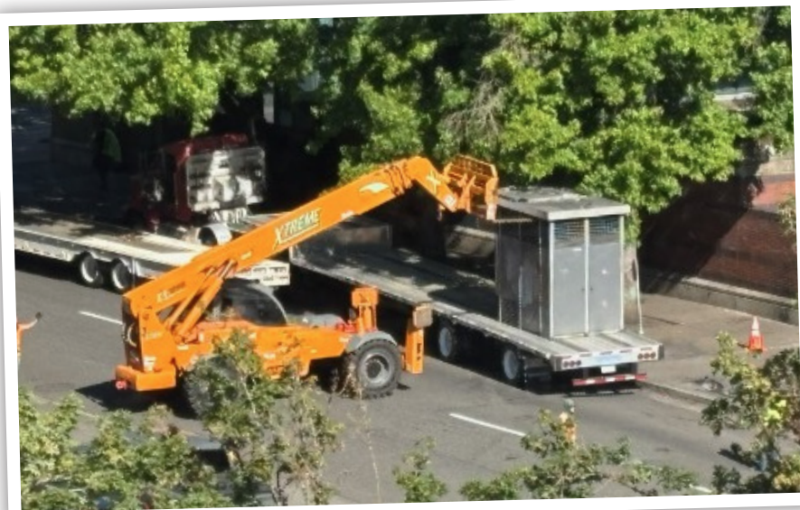
The Portland Loo at Northwest Fifth and Glisan streets was hauled away and won't be replaced. Installed in 2008, it was the oldest Loo in the city and beyond repair. TriMet recently purchased the former Greyhound terminal on that block and found the structure a barrier to access of the site. Portland Solutions approved of the removal.
