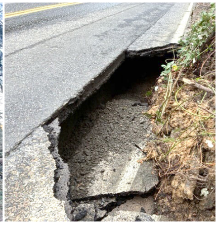
Cornell Road was closed for the last half of March due to a major landslide between the tunnels. Another mid-month landslide created a sinkhole under Cornell between Northwest Thompson and Skyline Boulevard, a section that remains closed.
