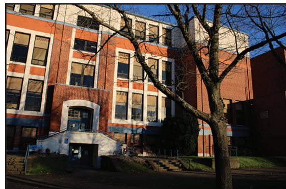
Portland Public Schools has planned to renovate and modernize Jefferson High School since 2012.
