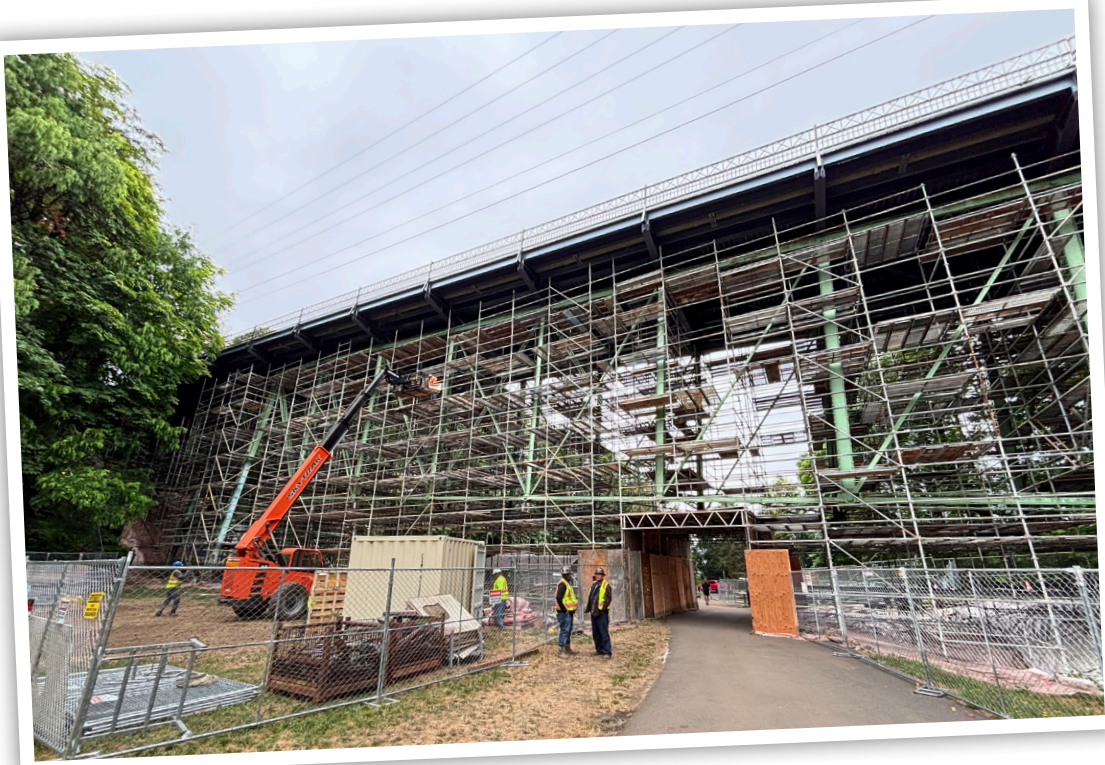
Scaffolding envelops the Thurman Street Bridge, which is being repainted and repaired and street lights added. About 70% of the $4.9 million project is covered by a federal grant. Buses and westbound traffic is detoured during the repairs.
