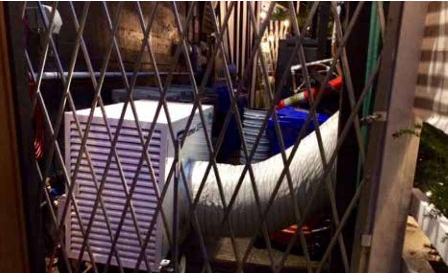
Café Nell's industrial-scale space heater generated noise far above the 55 decibel limit in residential zones, but Portland Noise Control Officer Paul van Orden deemed a temporary wall that cut the level to 57-58 dBA a sufficient solution.
