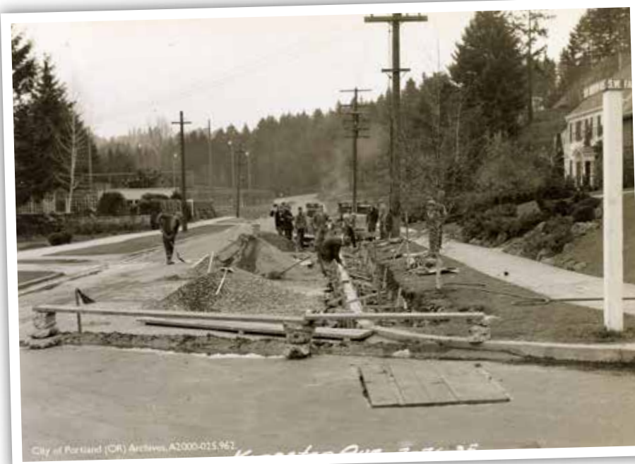
A crew repairs damage caused by a collapsed retaining wall at the intersection of NW Maywood Drive and Melinda Avenue in 1934.
