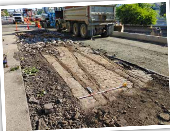
Streetcar rails buried under Northwest 16th Avenue for about a century were removed during construction of street improvements between Burnside and Davis streets. The Oregon Department of Transportation archaeology department documented the discovery and saved the materials. The Portland Bureau of Transportation will reuse the cobble stones on new projects. (Photo on left by Jacob Kovalchik, Archaeological Monitor)
