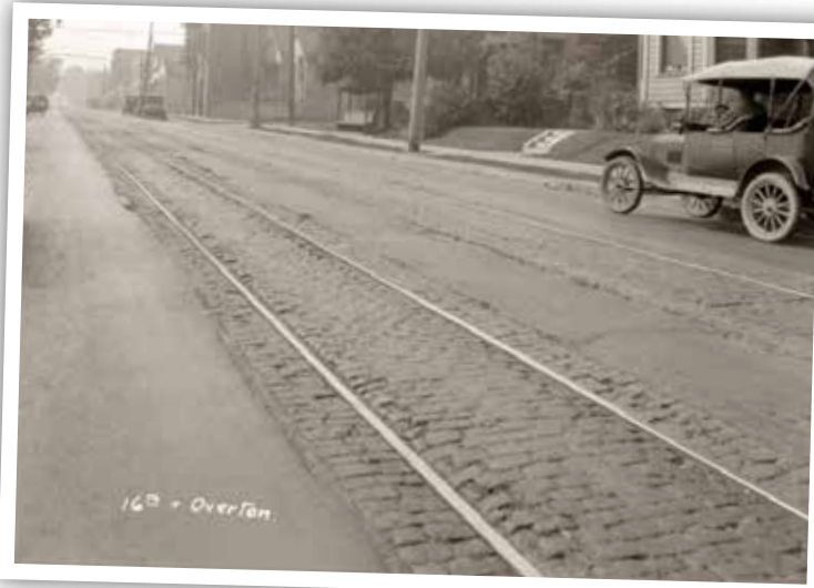
Streetcar rails buried under Northwest 16th Avenue for about a century were removed during construction of street improvements between Burnside and Davis streets. The Oregon Department of Transportation archaeology department documented the discovery and saved the materials. The Portland Bureau of Transportation will reuse the cobble stones on new projects. (Photo on left by Jacob Kovalchik, Archaeological Monitor)
